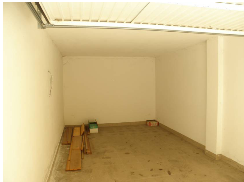
VISTA GARAGE PT
